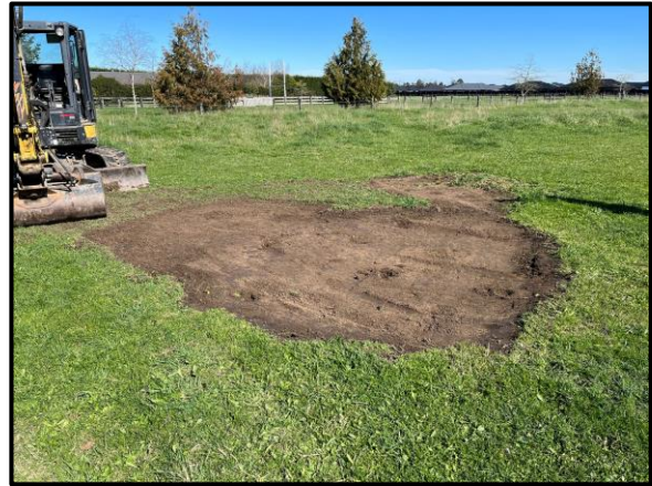
Photo 2: Remediated burn pile looking southwest
