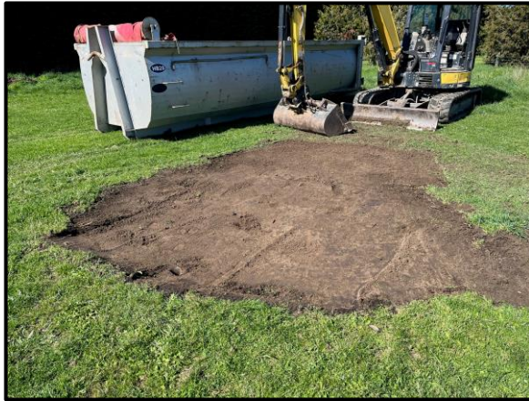
Photo 1: Remediated burn pile looking southeast
