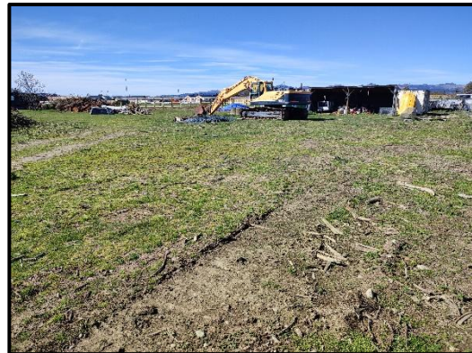
Photo 2: Sheds on east end of site
